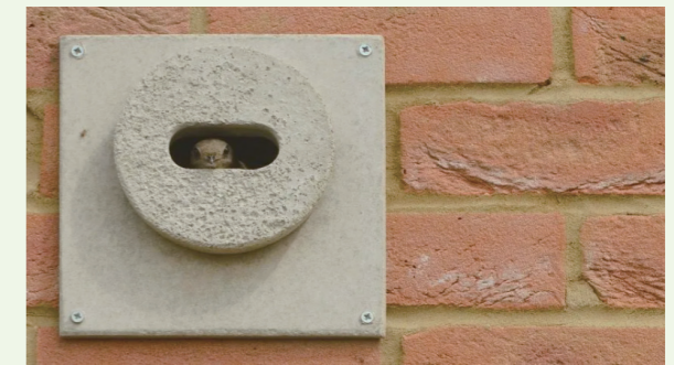
건물에 설치된 스위프트 브릭 출처: RSPB. (n.d.). Swift Bricks - we need action, not warm words. https://www.rspb.org.uk/whats-happening/news/swift-parliament-debate#the-swift-brick (검색일: 2026.3.10.)
