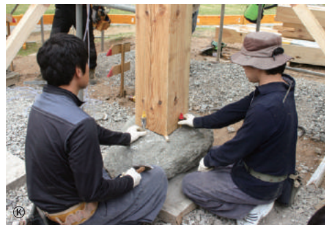
Checking verticality
