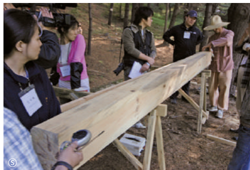
Marking the center line on a purlin
