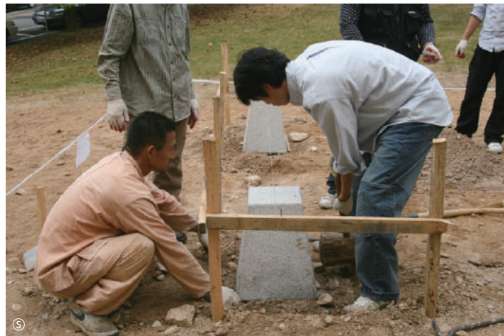
Placing column base stone
