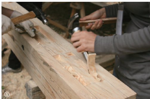
1 2 — 1 Placing the timbers on the workbench 2 Sawing joint 3 4 3 Carving mortises 4 Carving a groove on wall stud
