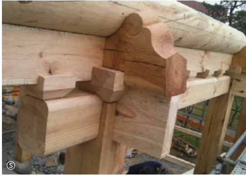
Joining method of columns, beams and purlins
