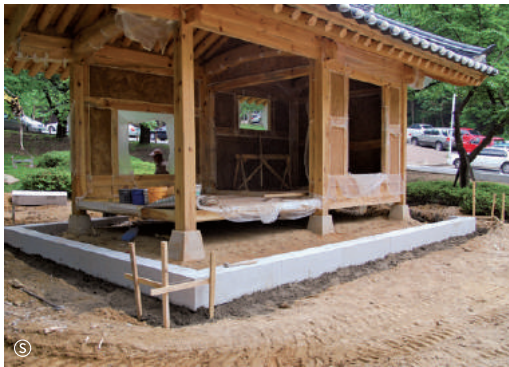
Placing border stones
