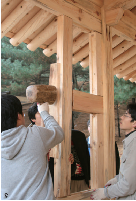
Assembling wall studs
