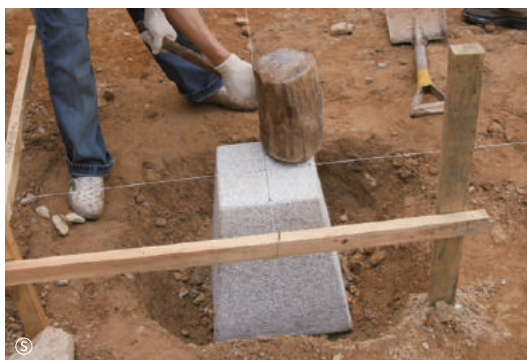
Laying the column base stone in the correct orientation
