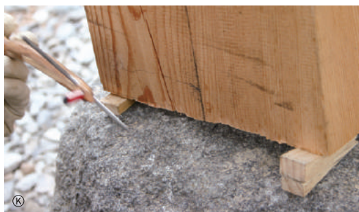
Fitting two components(column and base stone) for connection
