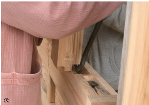
Assembling wall studs
