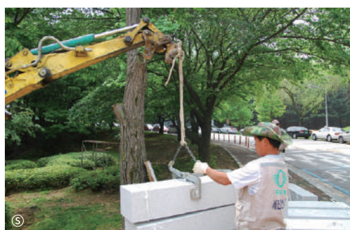
Lifting and carrying stylobate stone
