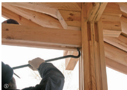
Assembling the upper lintel
