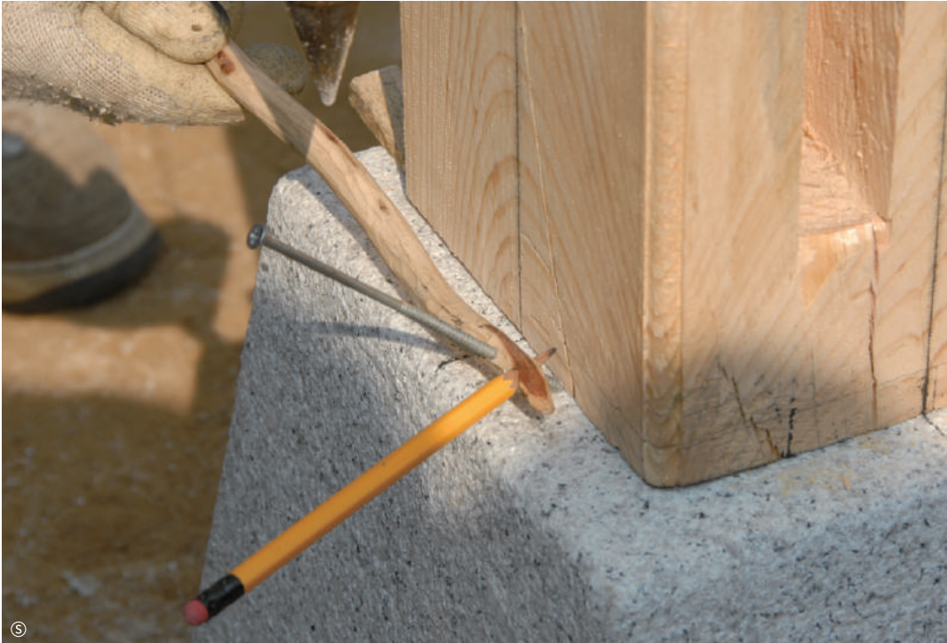
Fitting column base stone and column
