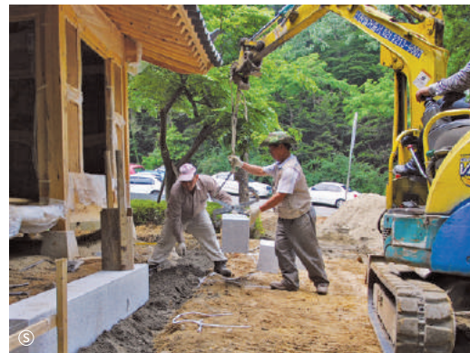
Placing border stones
