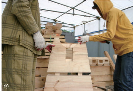
Joining the components of the flat truss post
