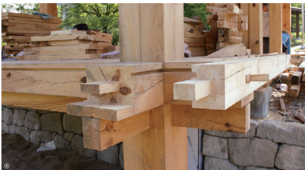
1 — 1, 2 Assembling floor joists 2
