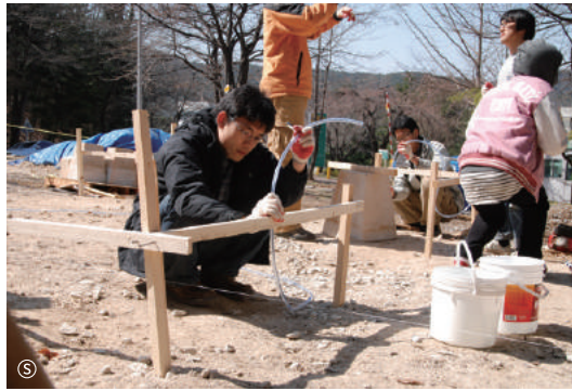
Using a water level
