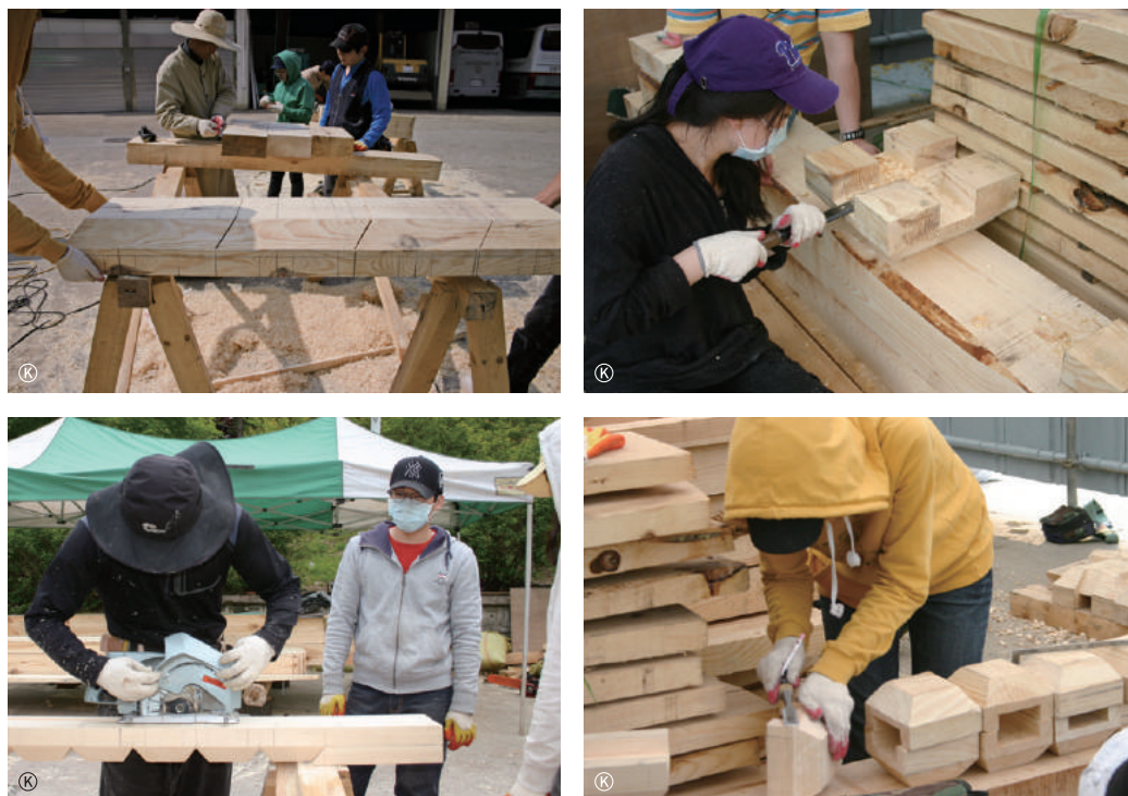
1 2 — 1 Marking and trimming capital 2 Carving dovetails 3 4 3 Trimming small bearing block 4 Chiseled work
