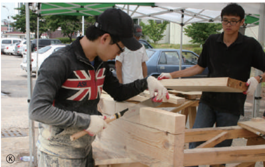
Trimming the protruding railing
