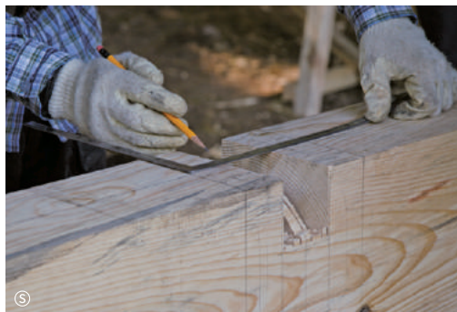
Marking and trimming purlin
