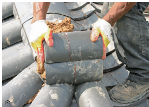
1 2 — 1 Laying roof ridge 2 Capping 3 4 3 Capping with a cover tile 4 Capping with a decorative tile
