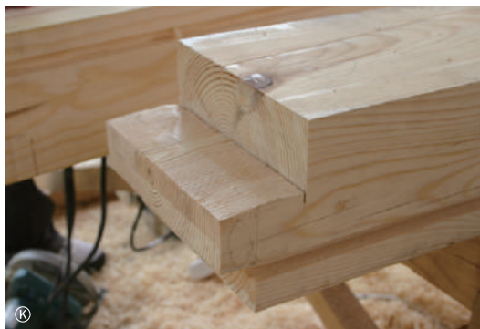
Carving a rabbet of the short floor joist
