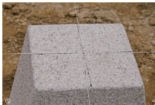
Marking the center of column base stone
