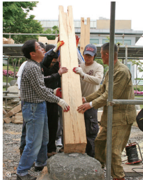
Erecting column
