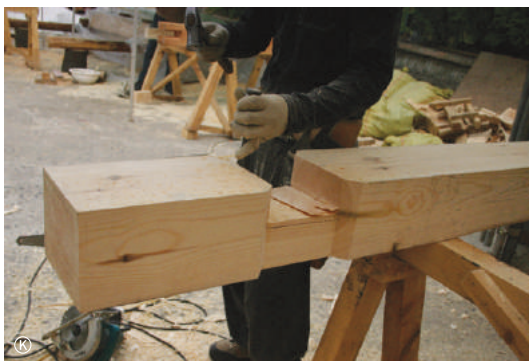
Carving mortises of the long floor joist
