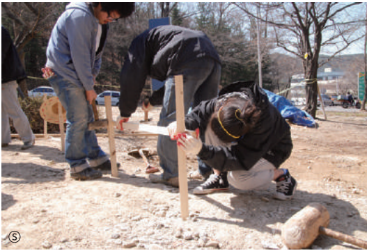
Placing batter boards
