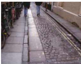
Granite kerbs and channels, settled carriageway and sandstone flag footway in laneway.
